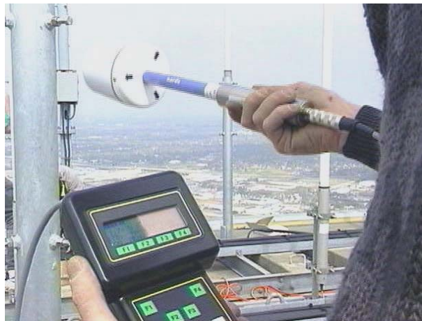
Figure 6. RF field measurements are routinely performed with broadband RF field probes and meters, as above, whenever changes in the operational environment occur.
