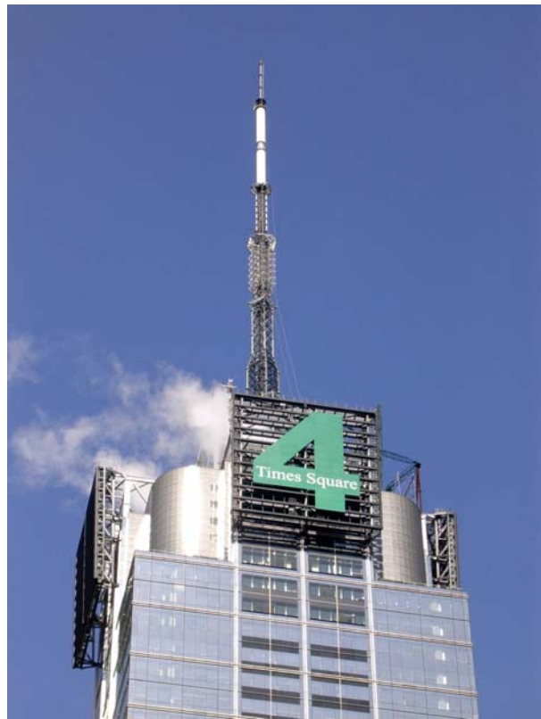
Figure 1. The 4 Times Square building showing the antenna mast with master antennas for FM radio and VHF and UHF TV broadcasting.
