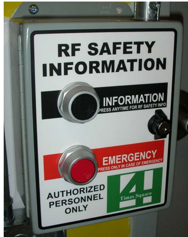
Figure 15. Close-up photograph of the TowerSwitch™ RF safety door enunciator unit that is mounted at main roof access doors, outside on the main roof, and at the hatch and door access points for the antenna tower.
